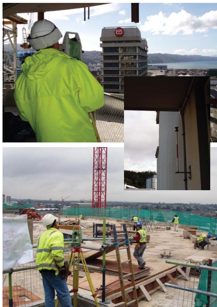
Figures 2, 3 and 4: Surveying part of the Wellington Regional Hospital building, with observations to prisms on surrounding buildings similar to that demonstrated
